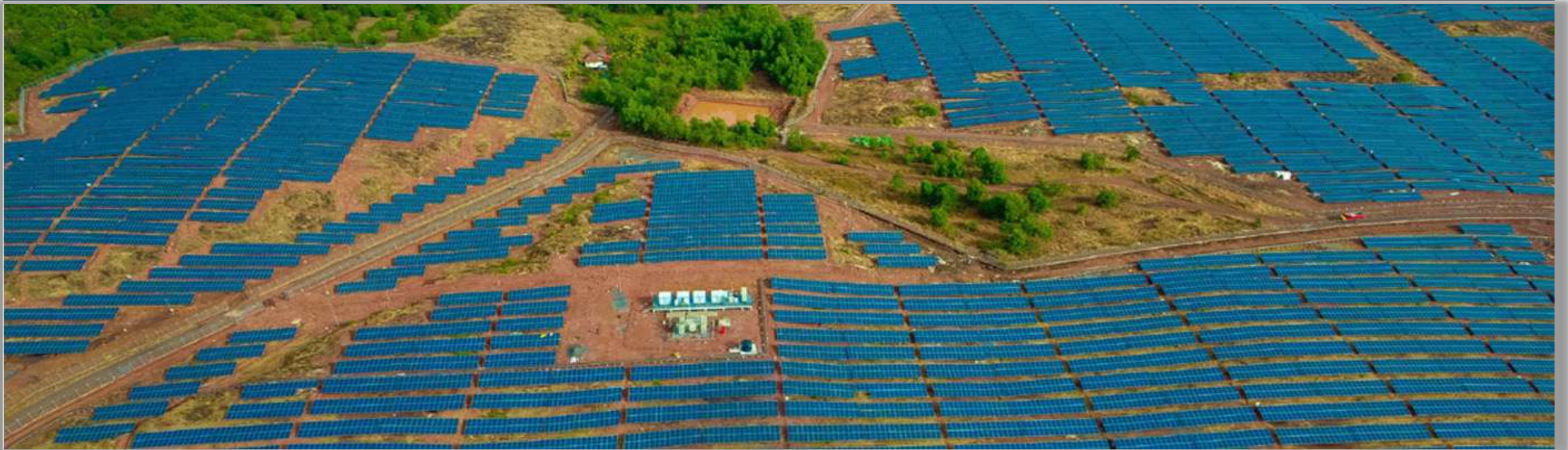
Aerial view of 50 MW solar plant at Kasargod under RPCKL
