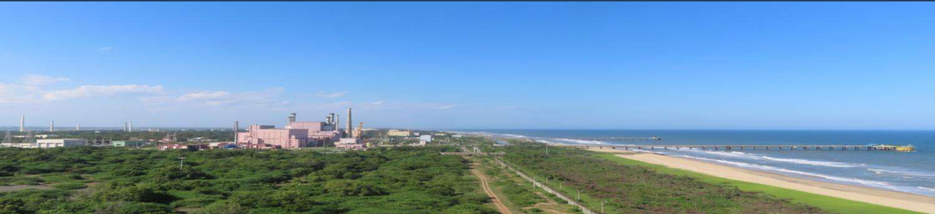
COASTAL SITE – PROTOTYPE FAST BREEDER REACTOR, KALPAKKAM, TAMILNADU
